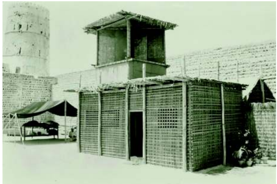
Figure 1.2d When additional ventilation is desired, wind scoops can be used, as on this reconstructed historical dwelling in Dubai. Also note the open weave of the walls to further increase natural ventilation. Although this is a desert area, lightweight construction is appropriate because the region along the Persian Gulf is humid. (Photograph by Richard Millman.)
